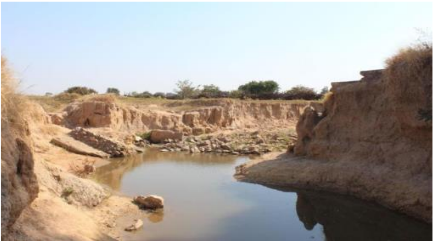
Total washaway of drop structure 3
