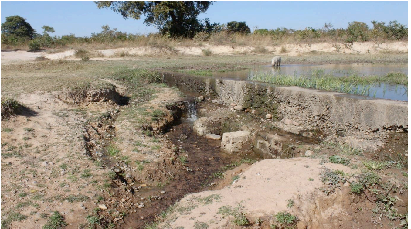
Figure 22: Erosion at Drop Structure 1
