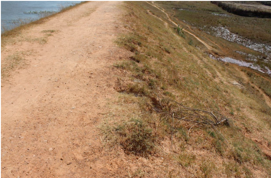
Downstream crest showing breakaway and gully formation
