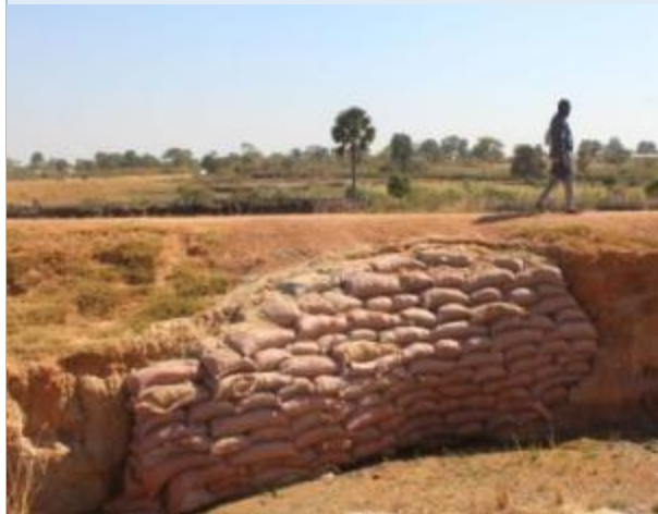
Photo Spillway channel training wall repaired by the local community
