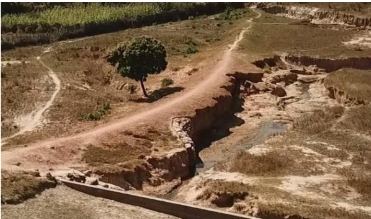
Spillway erosion
