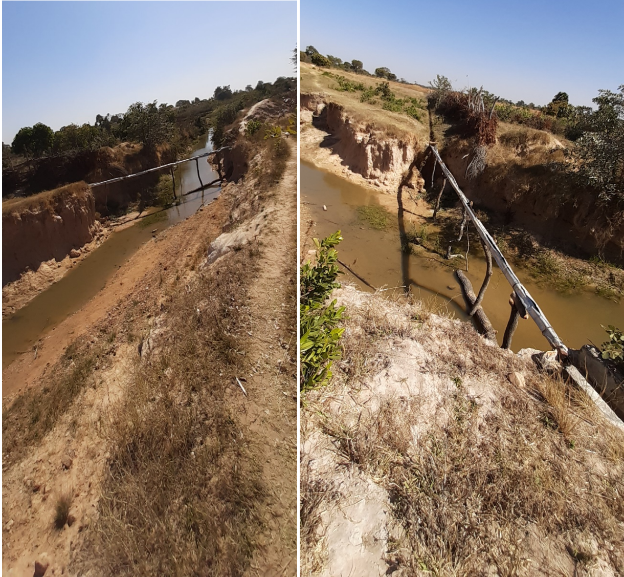
Figure 29: Broken canal over channel due to expanding eroded return channel- temporarily fixed using logs
