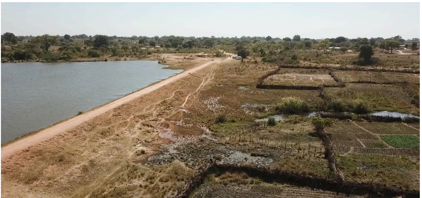
Seepage at toe and downstream to the river line
