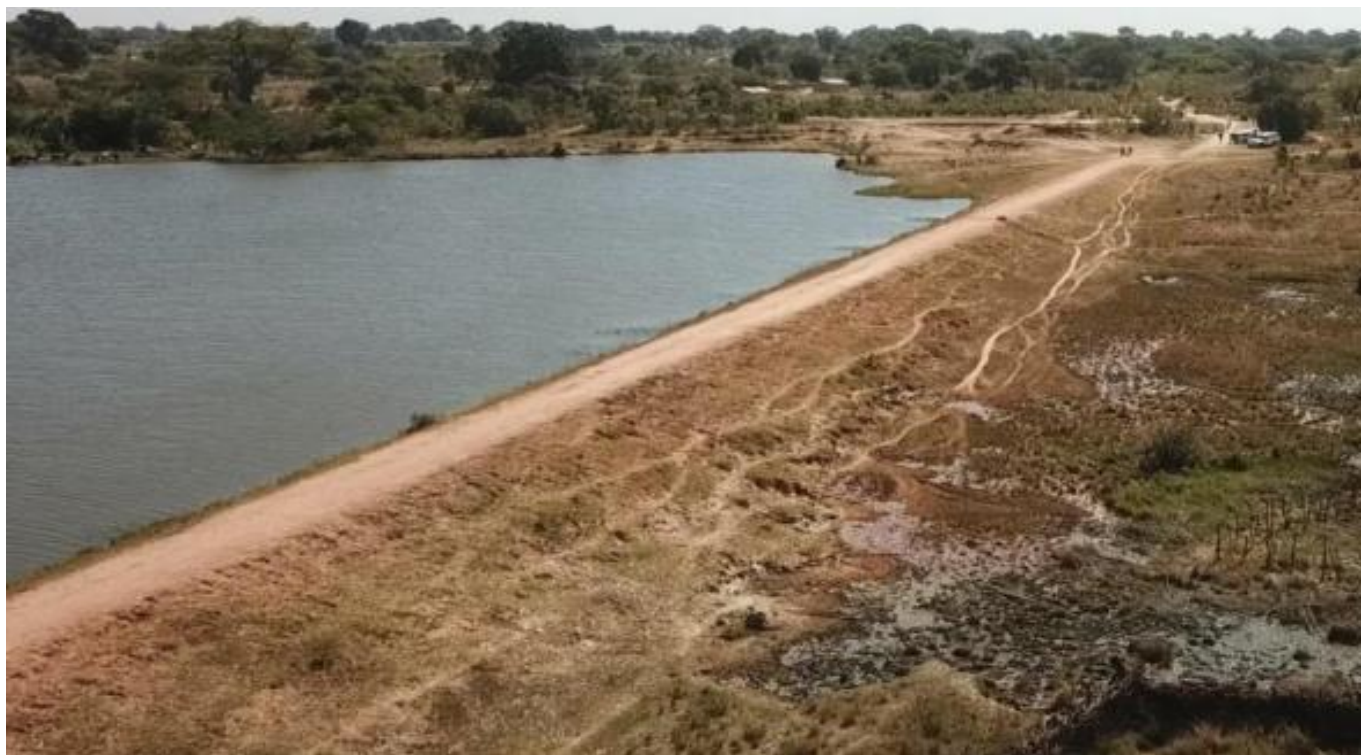
Seepage at and downstream of toe
