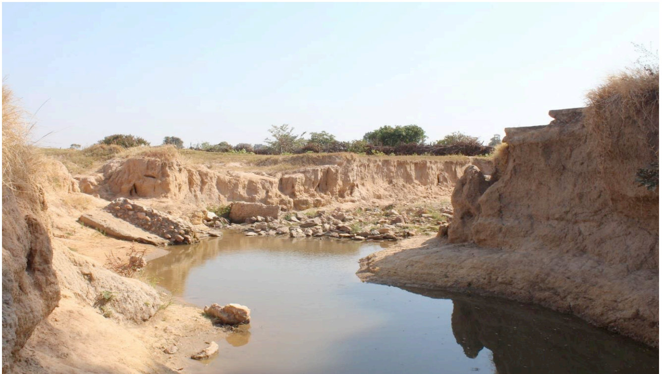
Figure 23: Total washaway of drop structure 3
