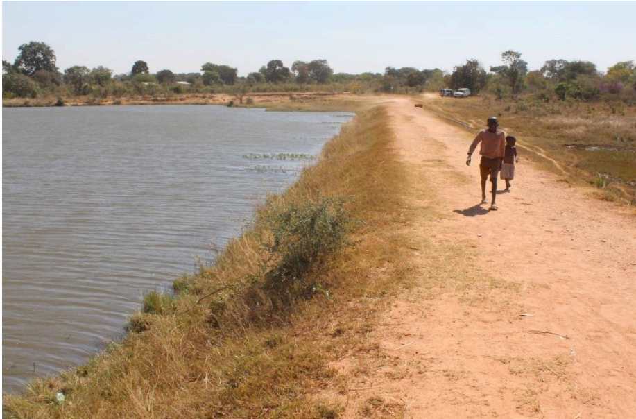
Typical condition of main embankment crest
