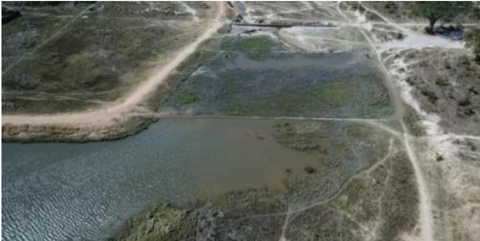
Service spillway and discharge channel – badly compromised effective width
