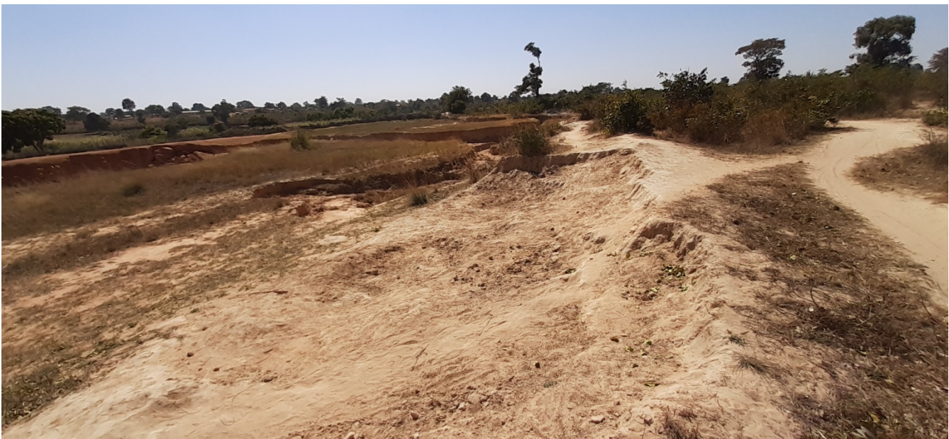
Figure 2: Open slopes and gullies along spillway and towards embankment
