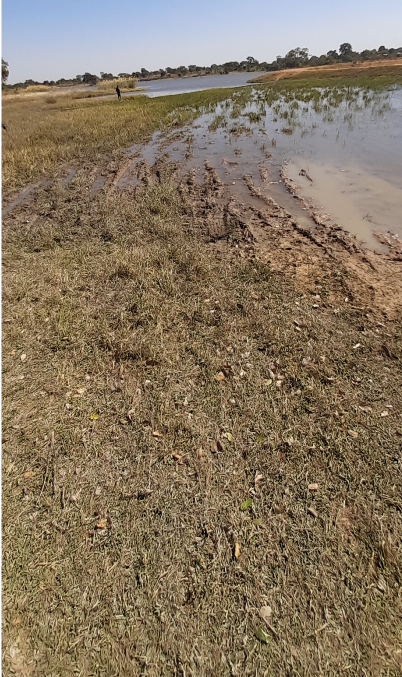
Figure 26: Pedestrian, livestock and ox cart road flooded at spillway going towards embankment (Ox cart tracks present)
