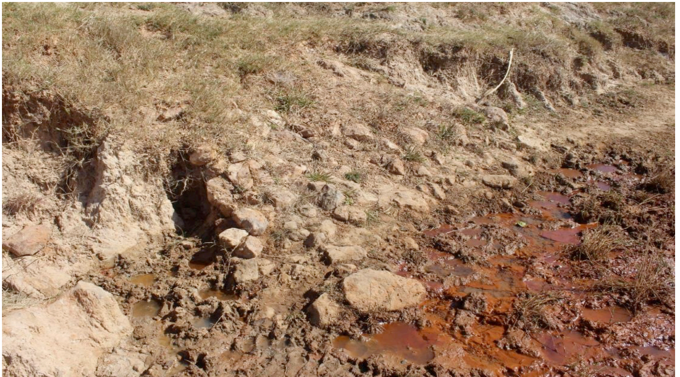
Figure 19: Seepage wet spot near rock toe location
