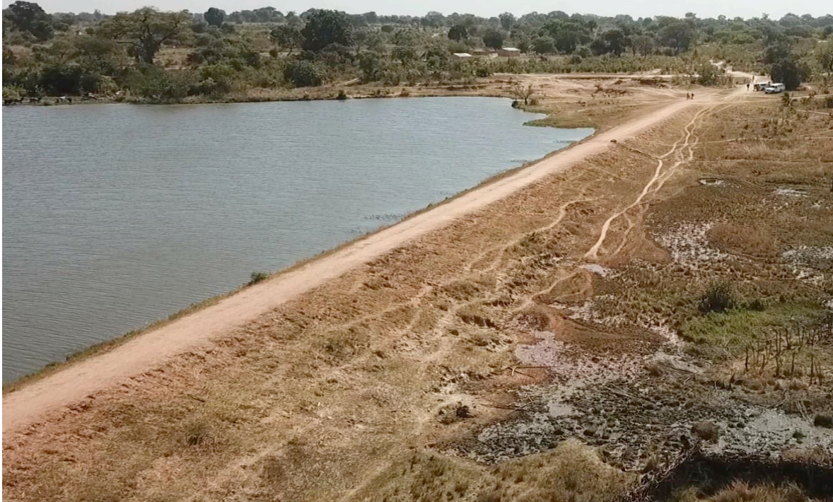
Downstream face of embankment - gullying and livestock footpaths
