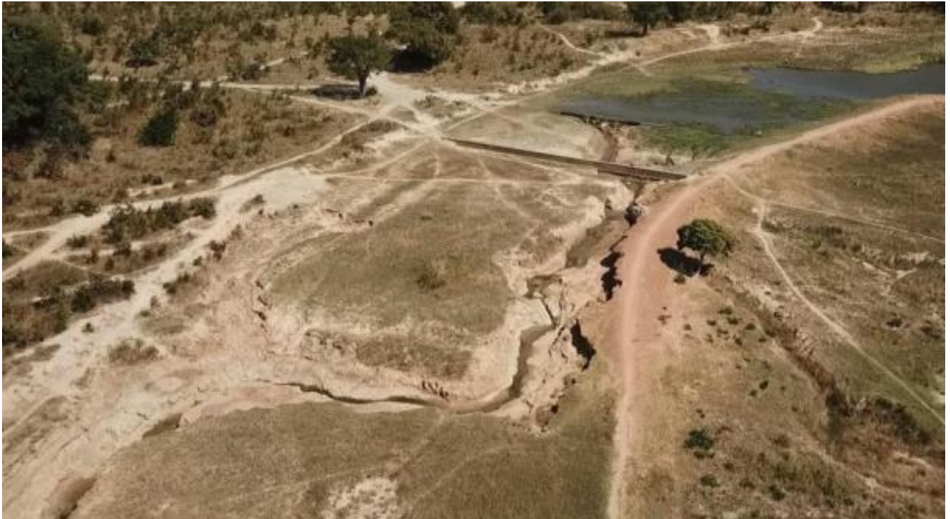
Spillway return channel showing drop structures, gully and training wall washaway
