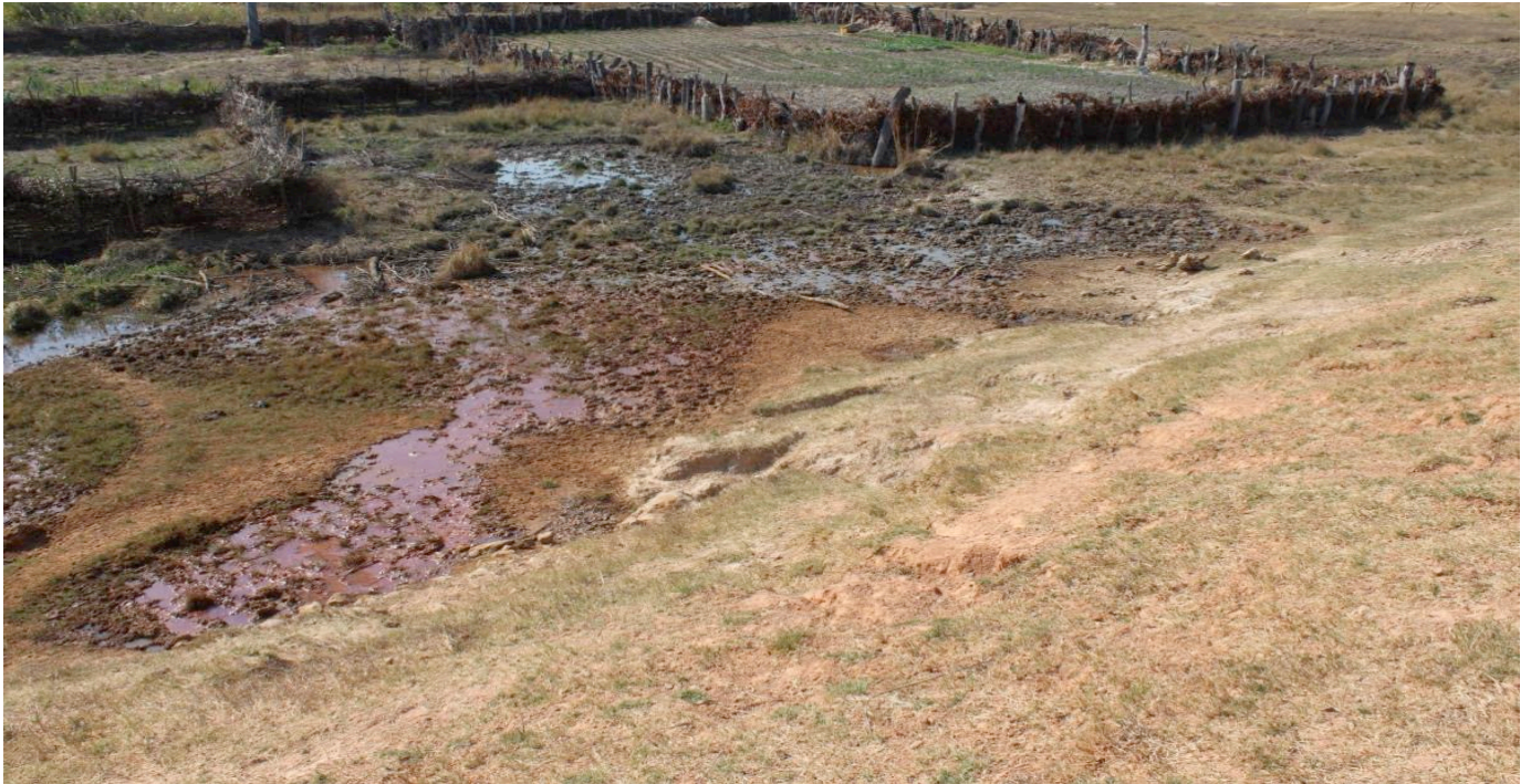
Seepage at rock toe and right flank of river
