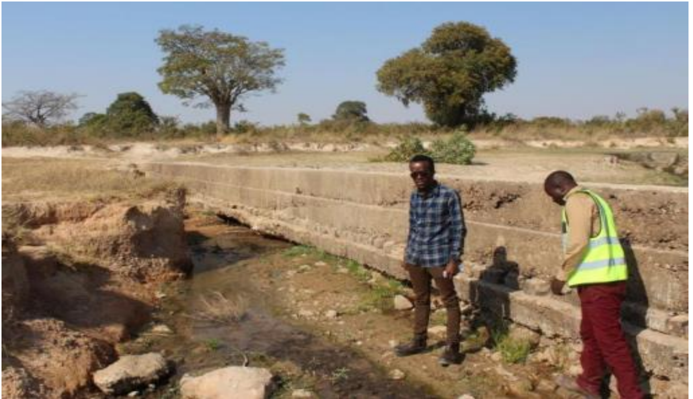
Erosion at drop structure 2
