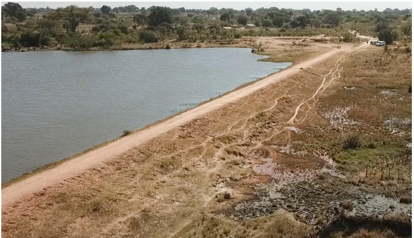
Figure 21: Seepage at and downstream of toe and livestock paths
