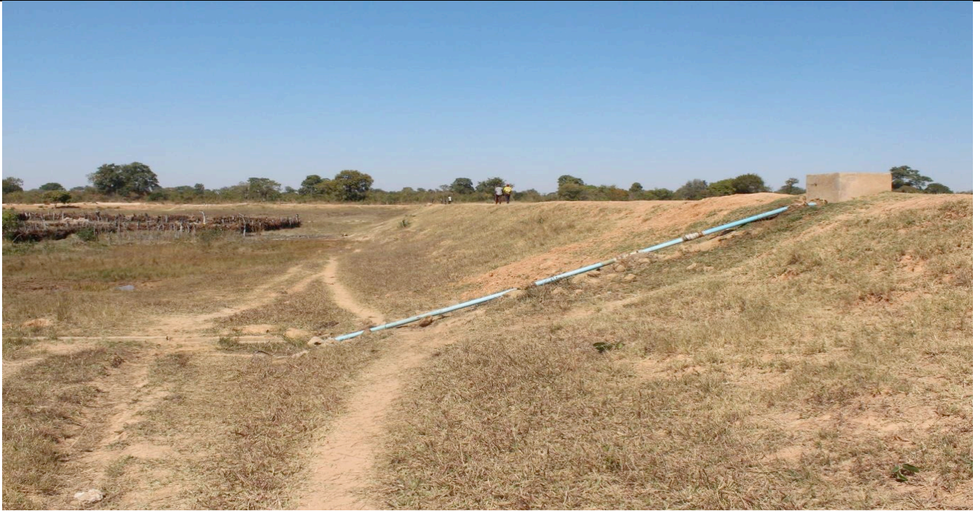
No evidence of toe drain on left flank
