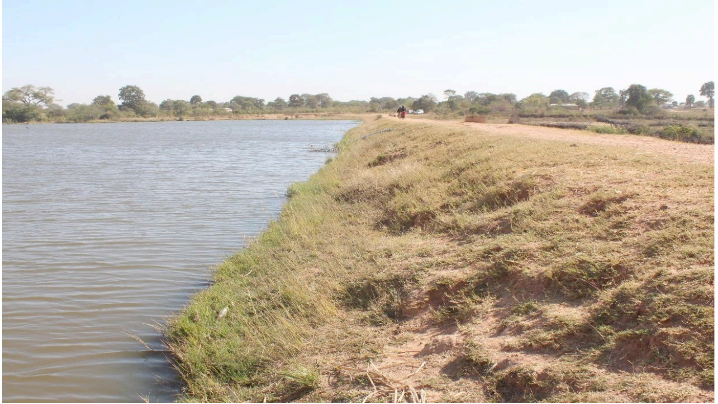
Figure 18: Front face condition requiring slope works
