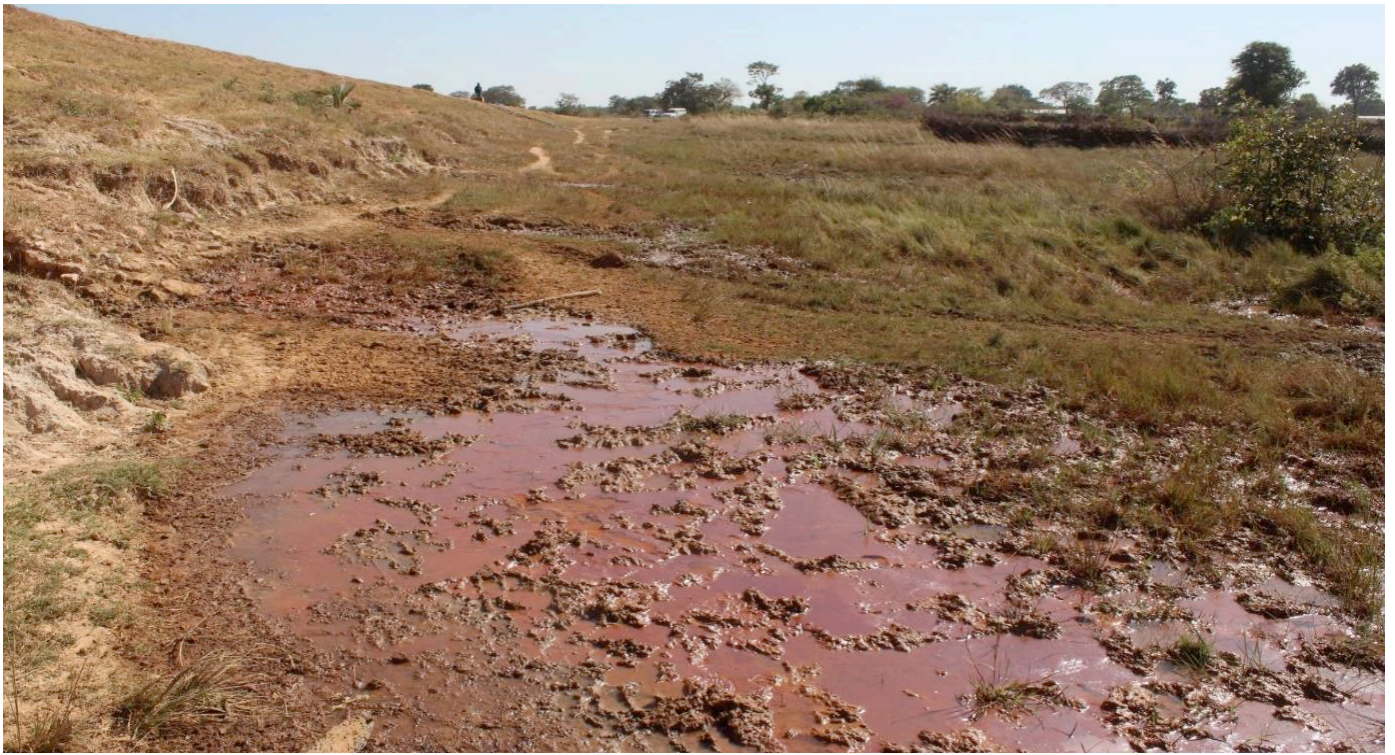
Seepage wet spot near rock toe location
