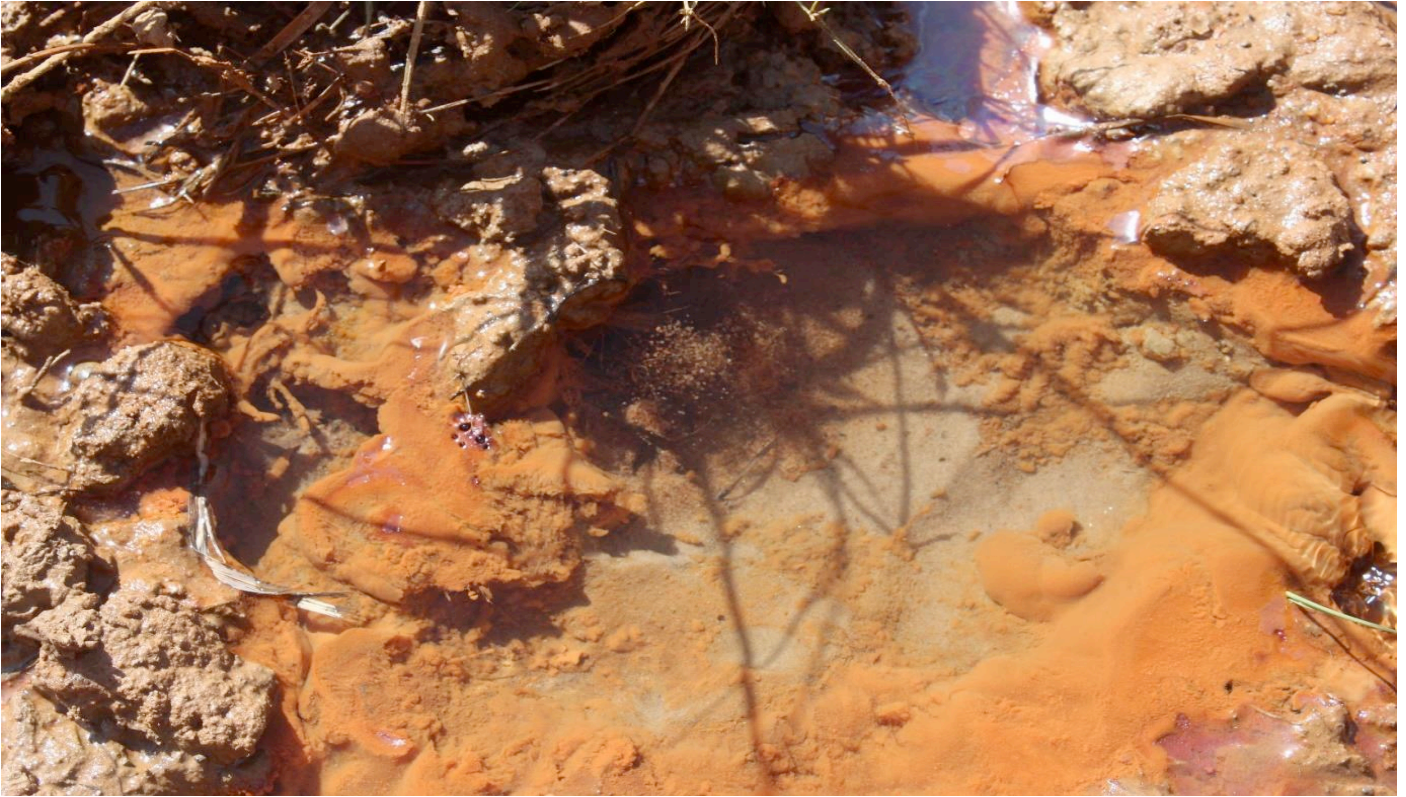
"Boil" evident in seepage near rock toe
