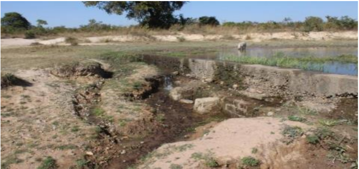
Erosion at drop structure 1
