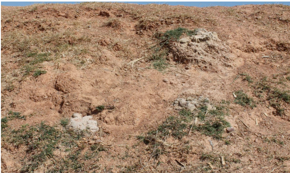
Termite workings partially blocked with cement
