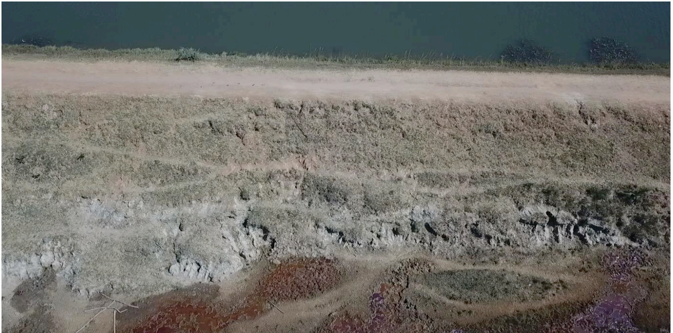
Aerial view of seepage along toe of embankment
