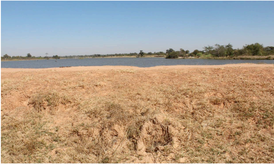
Termite workings on downstream face near crest
