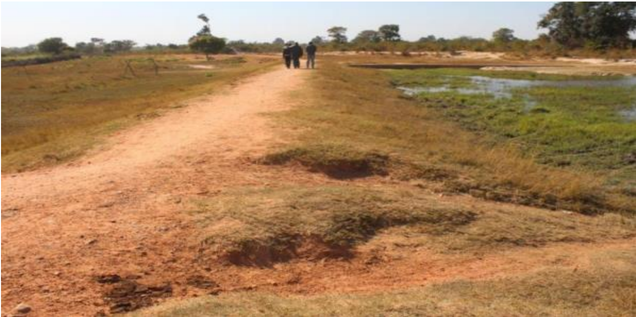
Embankment end at spillway sill showing erosion damage
